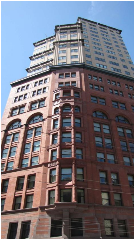
Built in 1890 as The Chronicle 's home, the De Young Building at 690 Market St. has gone through a procession of changes, including a 30-plus-year interval where its walls of sandstone and brick were clad in porcelain, aluminum and glass. The modern wrapping was removed in 2007 as it was converted to condos. To defray the costs, the owner was allowed to add extra floors to the building. John King / The Chronicle
